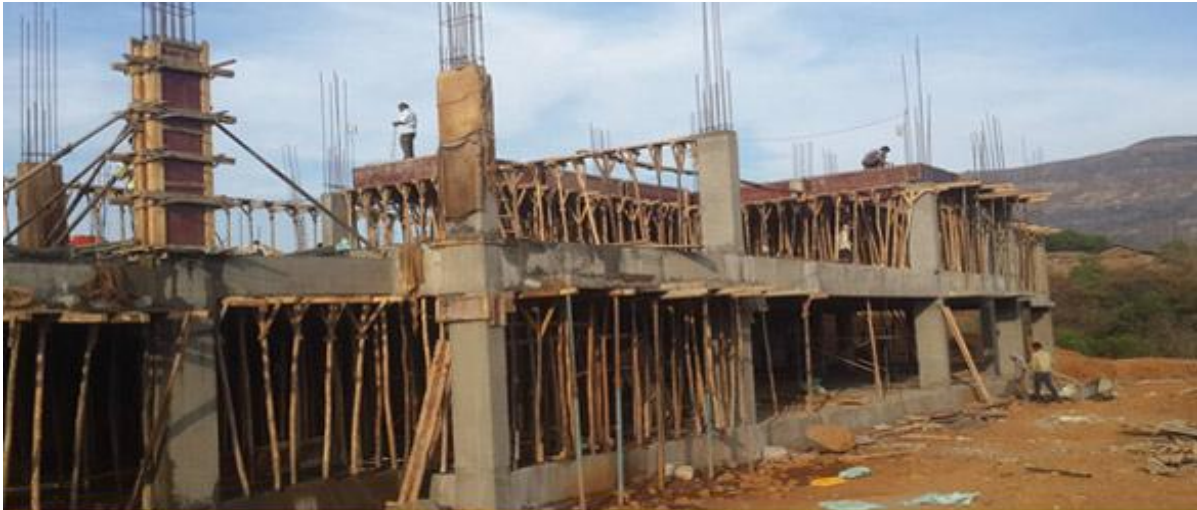
Construction Work is underway at Igatpuri
